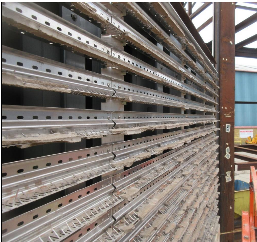
TEST SAMPLE DURING DISMANTLE
