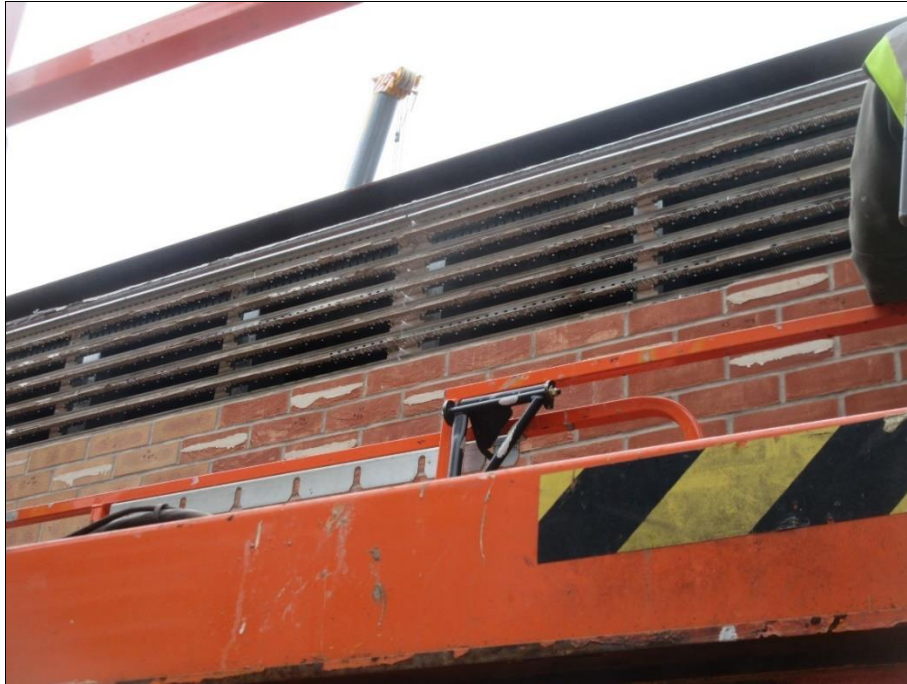
TEST SAMPLE DURING DISMANTLE
