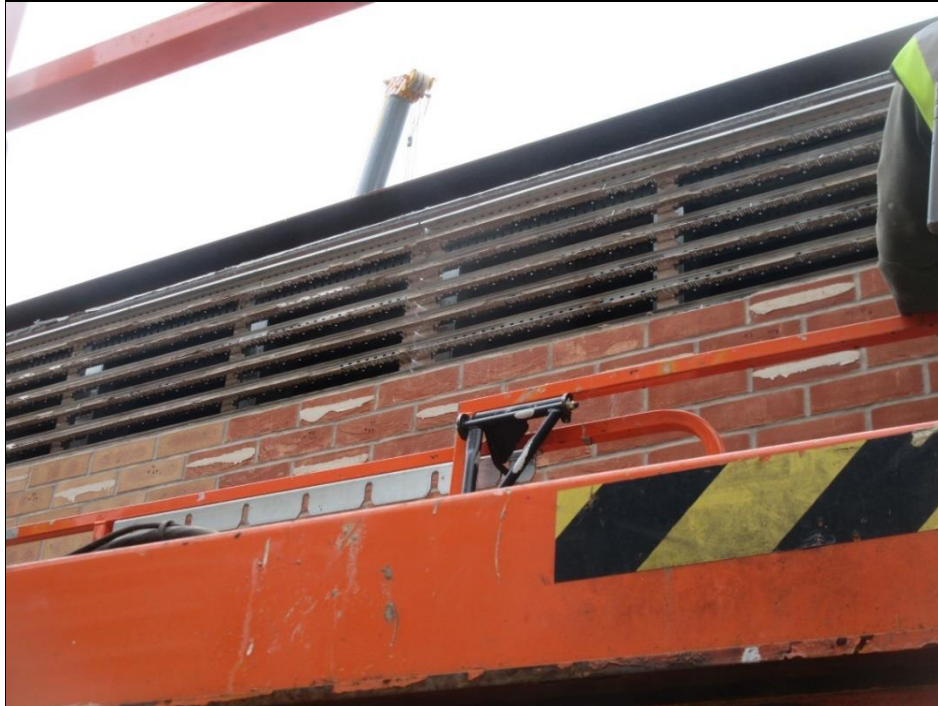
TEST SAMPLE DURING DISMANTLE
